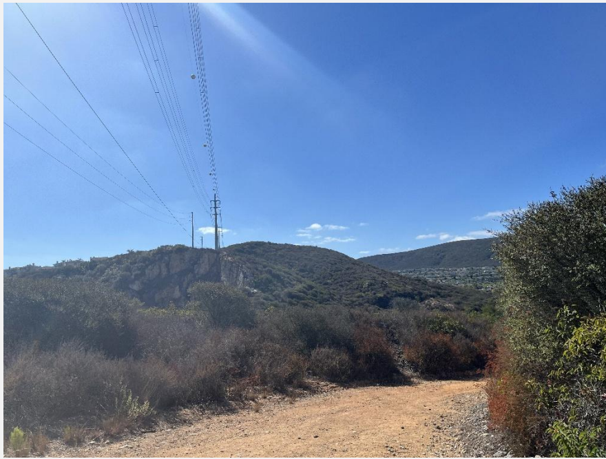
Photo 27. Photo Location 6 looking south
