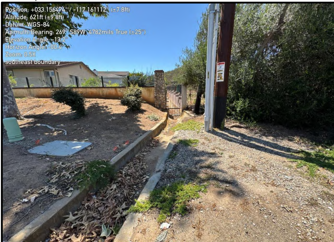
Photo 16: This concrete lined channel forms part of the southeast boundary, just off-site, and drains west to east under Twin Oaks Valley Rd.
