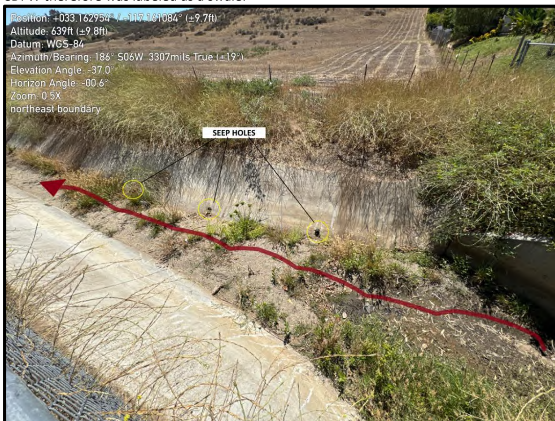
Photo 14: A wide concrete channel is located just northeast outside the project boundary. The channel funnels water from off-site north to south, eventually draining east under Twin Oaks Valley Rd.
