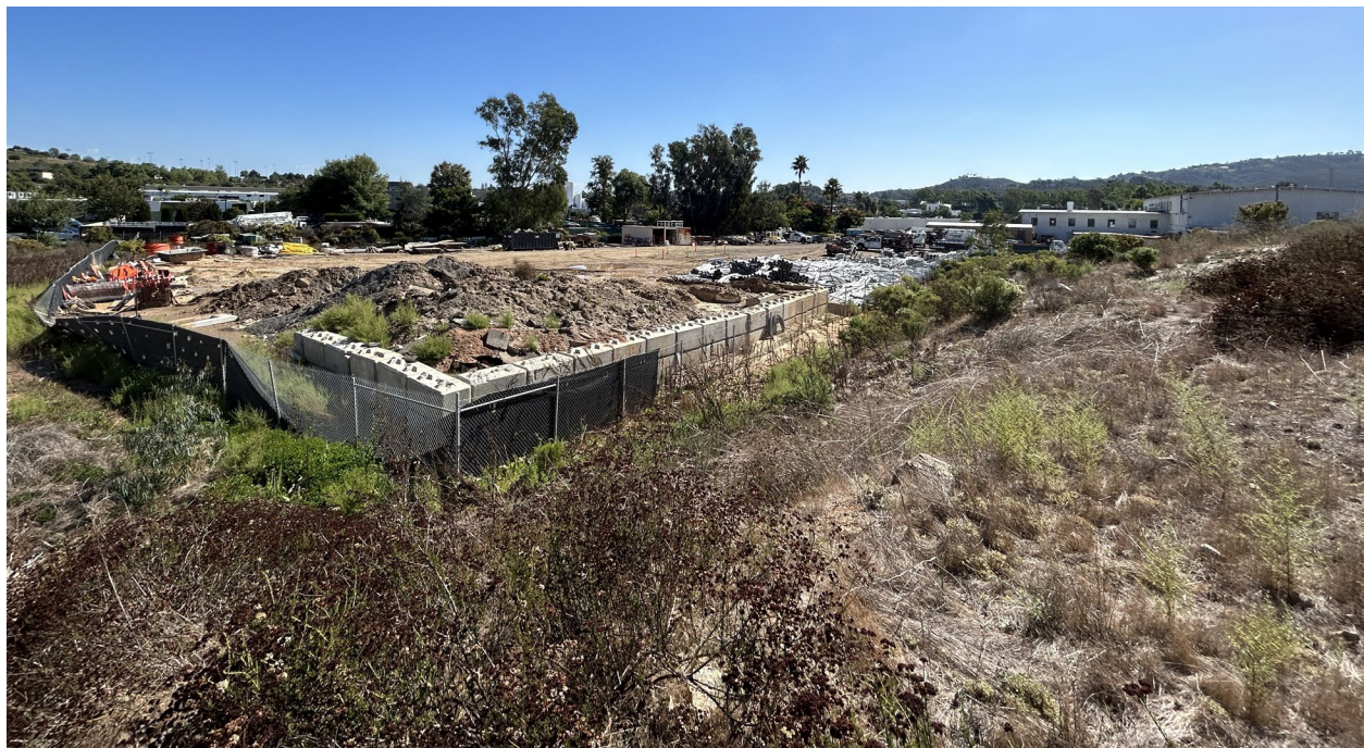
Figure 3. Overview of the existing conditions at the Project site, taken looking southeast from the top of the undeveloped slope in the northwestern portion of the site. The majority of the site is flat, with existing buildings visible in the background to the right.
